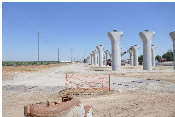
Picture 5: Ongoing construction at Kings/Tulare HSR station
