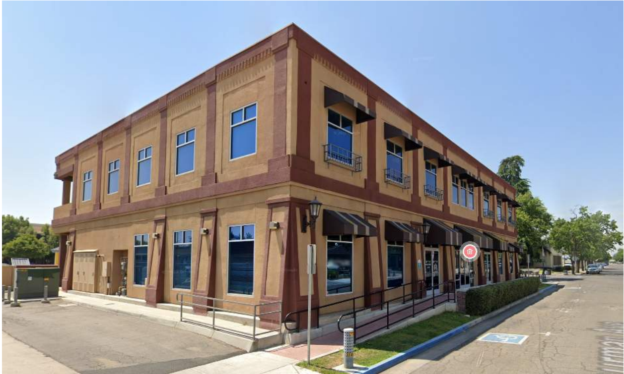
Photo 1: Centennial Plaza – Northwest Corner
