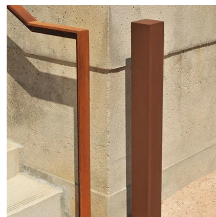
Corten steel railing and detailing throughout the site
