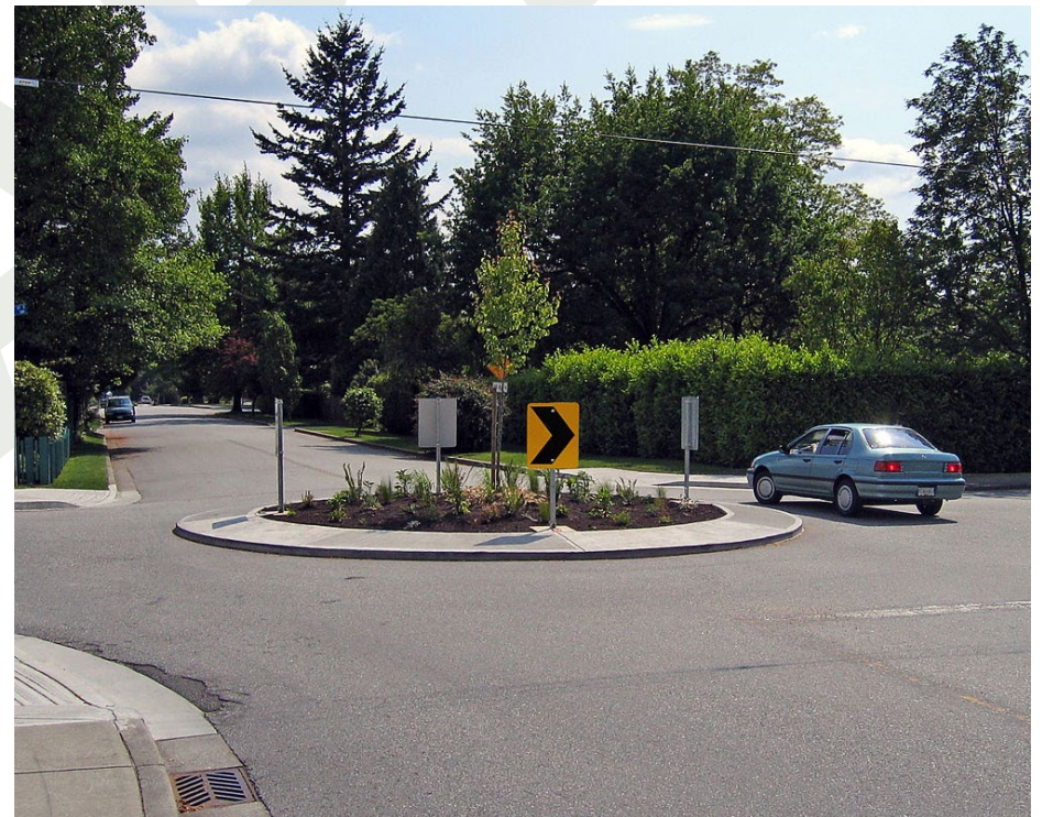
A traffic circle or roundabout is a form of circular intersection in which traffic travels counter-clockwise around a center island and entering traffic must yield to circulating traffic.
