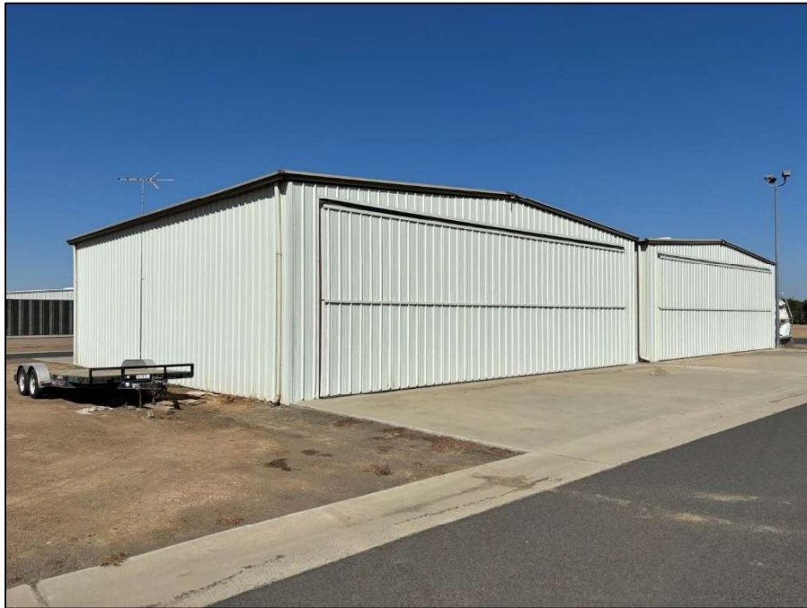
Exterior view of some small hangar ground lease parcels that have been improved with private hangars.
