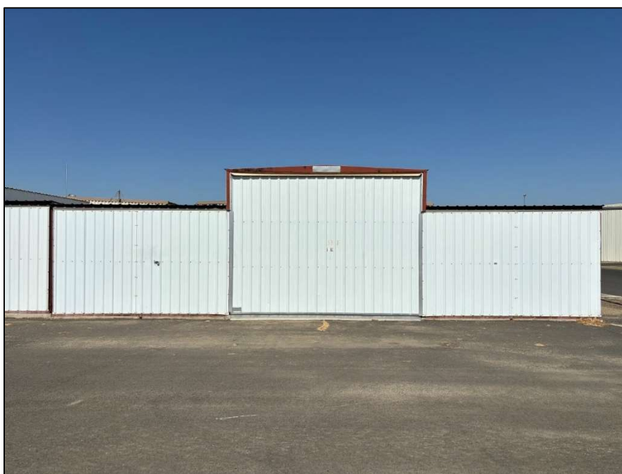
Exterior view of a typical city-owned T-hangar.
