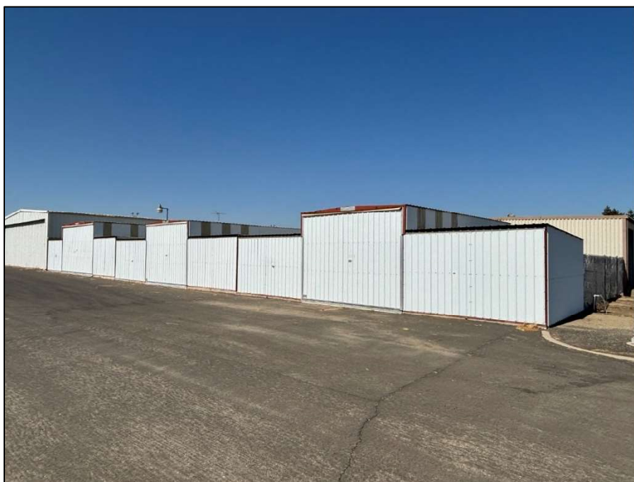
View of city-owned T-hangars.
