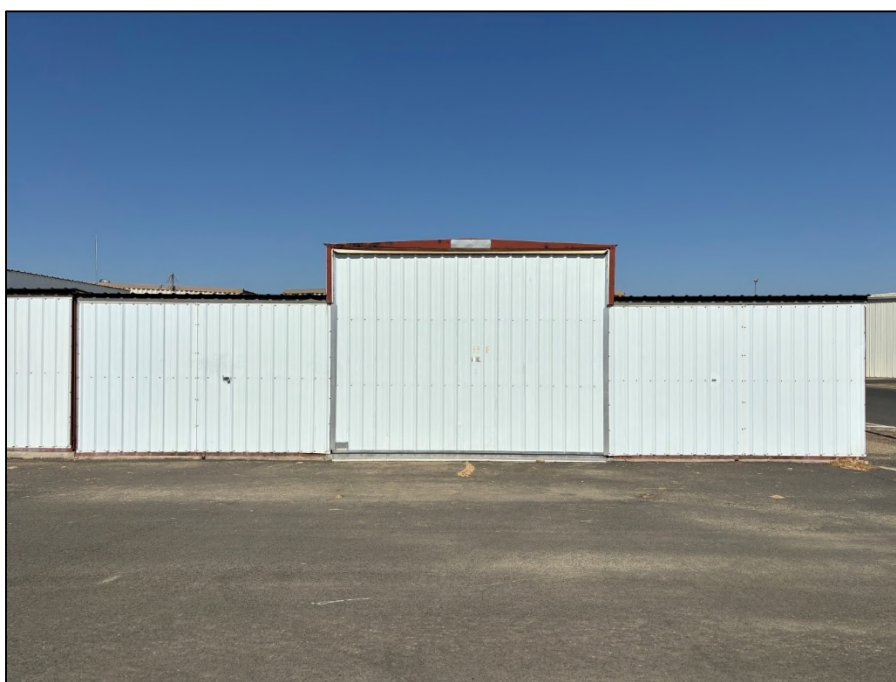
Exterior view of a typical city-owned T-hangar.
