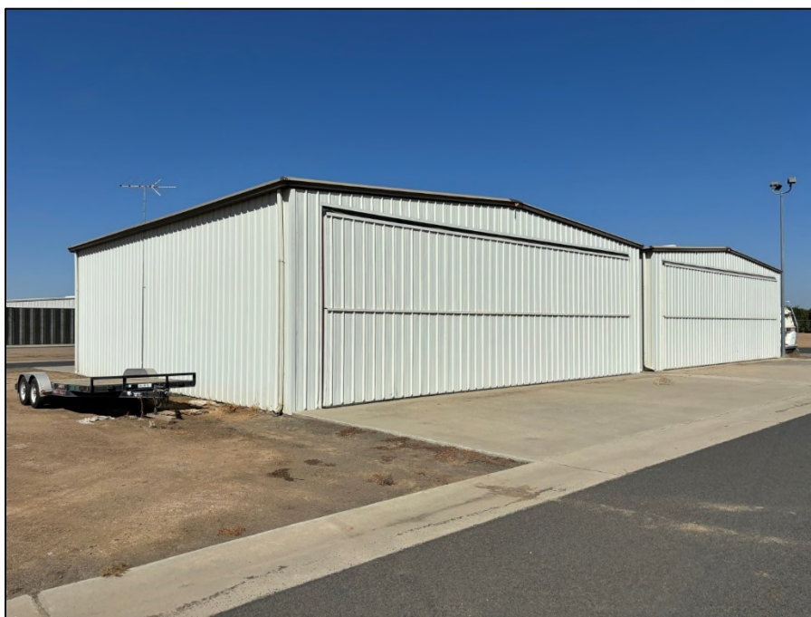
Exterior view of some small hangar ground lease parcels that have been improved with private hangars.
