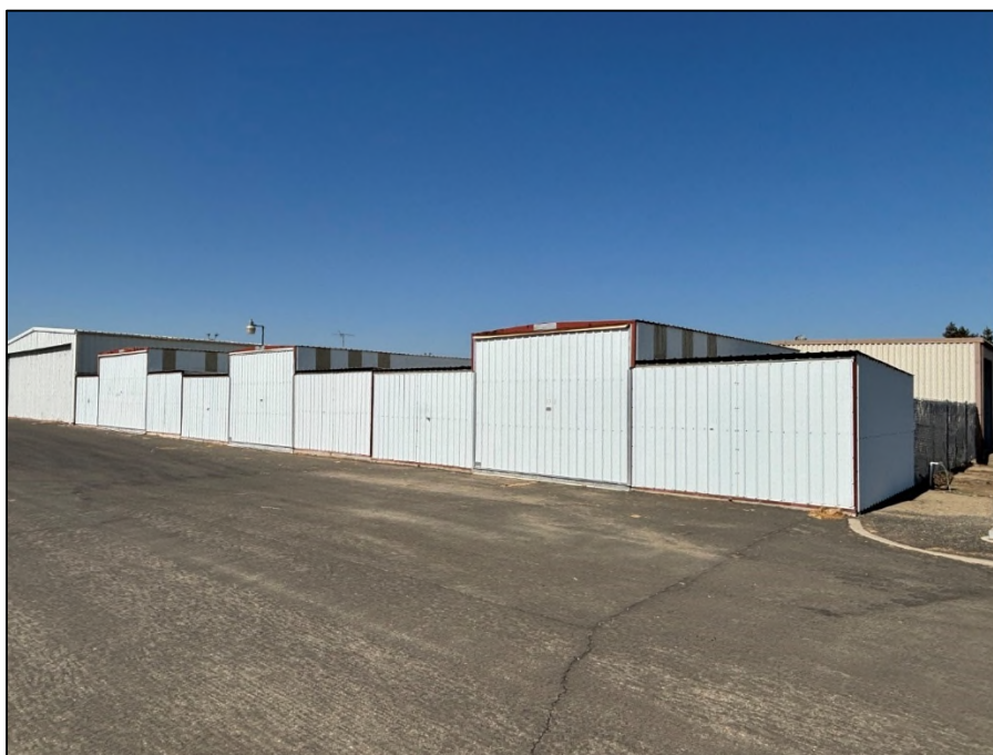
View of city-owned T-hangars.
