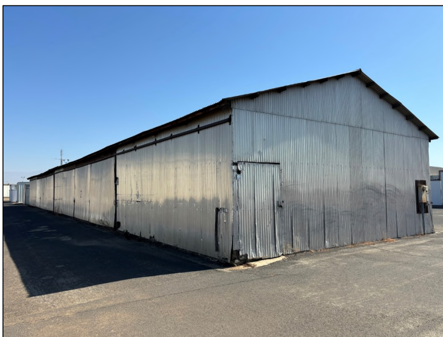
View of the city-owned hangar building on lot 32-A.
