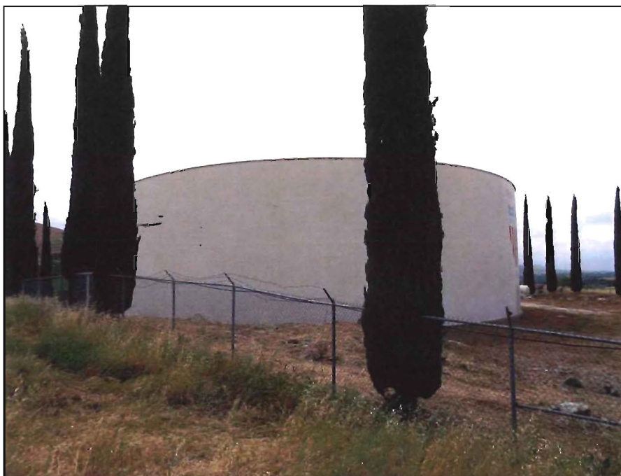
View of the existing tank site looking south from the new take area.
