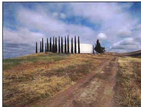
View of the subject property and the existing tank site along the dirt access road.
